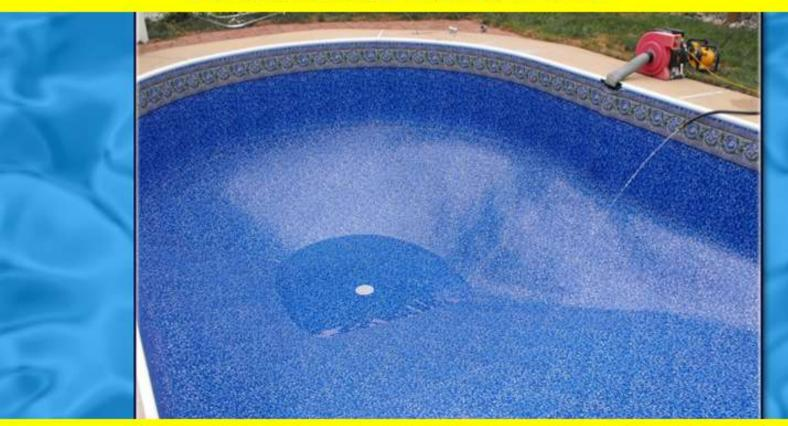
**VACUUM REMOVES AIR & KEEPS LINER WRINKLE FREE**
